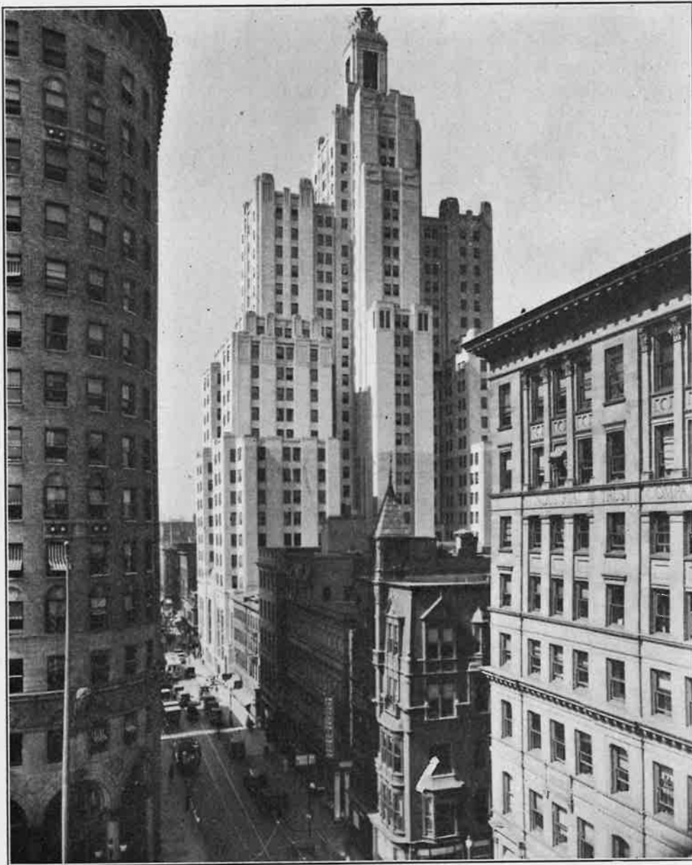
A STRIKING PICTURE OF THE "CANYON" THAT IS GROWING IN THE MIDST OF THE PROVIDENCE BUSINESS SECTION. A VIEW OF WESTMINSTER STREET, SHOWING THE NEW INDUSTRIAL TRUST BUILDING IN THE BACKGROUND, WITH THE TURKS HEAD AND OLD INDUSTRIAL TRUST BUILDING IN THE FOREGROUND.
